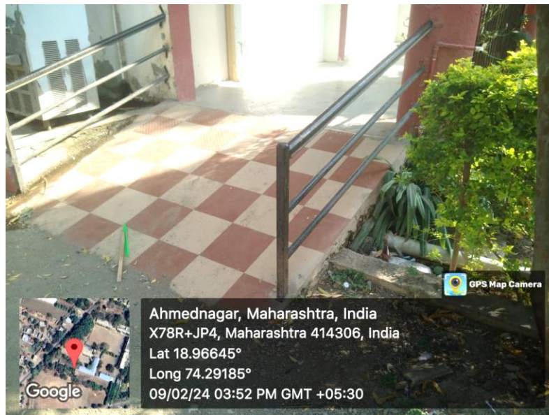
Photograph of Ramp for (Divyangjan) students to easy access to classroom
